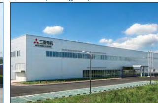
Mitsubishi Electric Automation Manufacturing (ChangShu) Co., Ltd. Programmable controllers, display panels (HMI), AC servo CNCs
