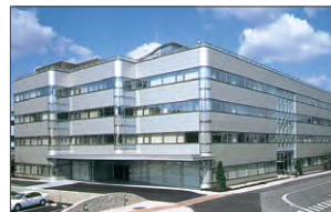
⑤Nagatsugawa Works Pressurized ventilators
