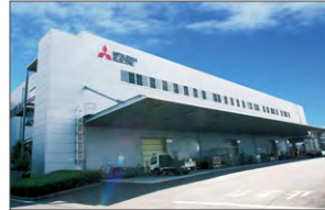
②Kani Factory Electromagnetic switchgear
